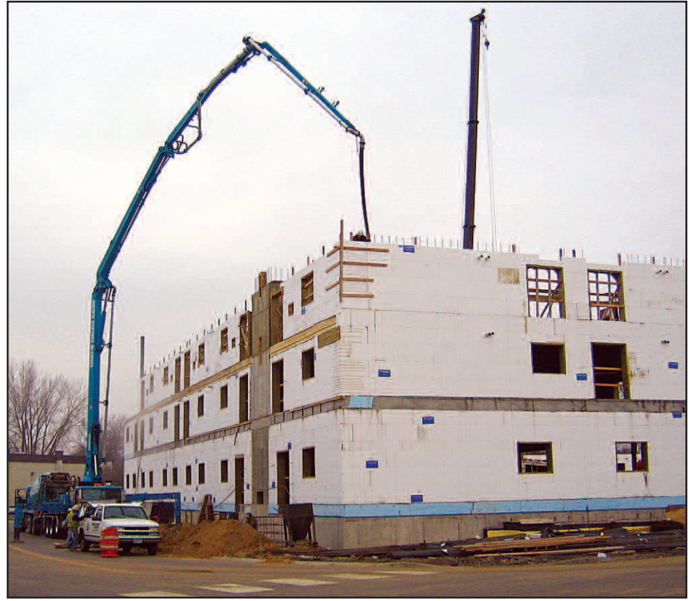
Crews pump the concrete into ICFs on the third story.
